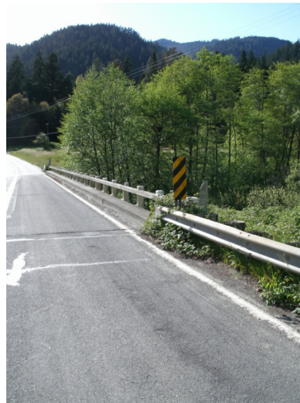
Figure 3 – West end bridge existing conditions, potential pedestrian bridge location
