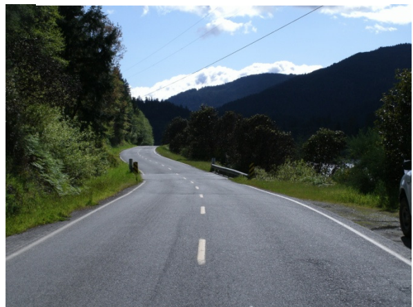
Figure 2 - Rough and Ready Bridge on Red Cap Rd.
