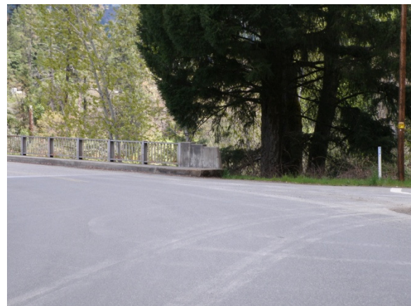
Figure 3 – Existing pedestrian facilities on bridge
