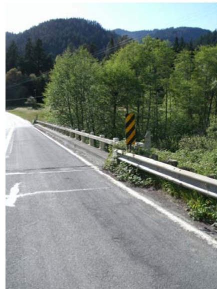
Figure 3 – West end bridge existing conditions.
