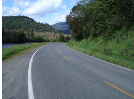
Figure 1 – Red Cap Road curvature, looking toward SR 96
