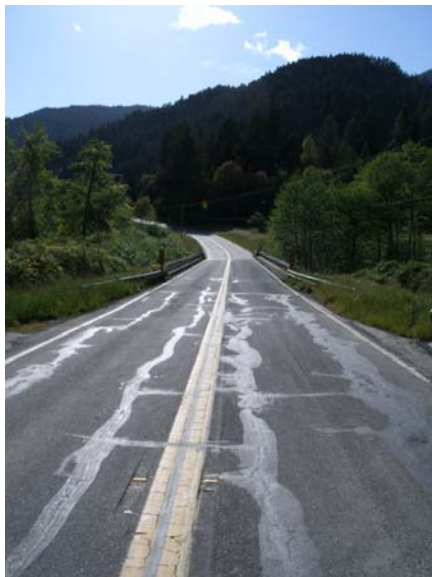
Figure 2 – West end bridge existing conditions.
