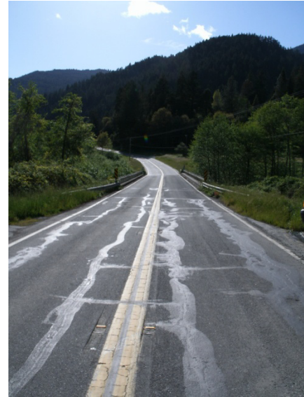
Figure 1 – Existing bridge west of Lower Camp Creek Road
