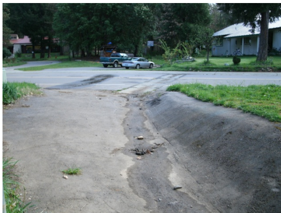
Figure 1 – Existing crossing facilities
