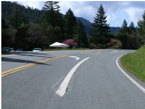
Figure 1 – Current striping, viewed from SR 96 south of intersection
