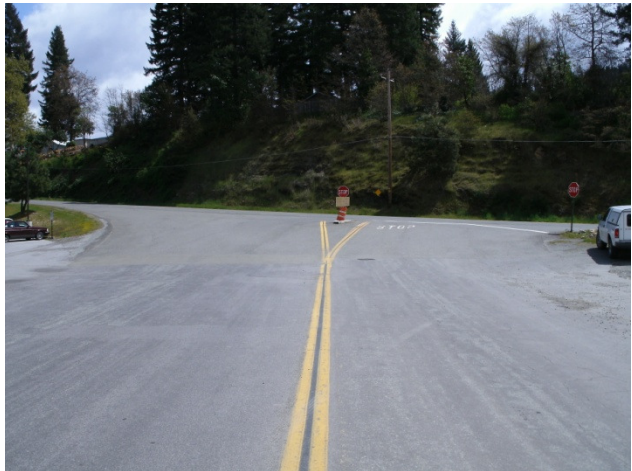
Figure 1 – Intersection looking east
