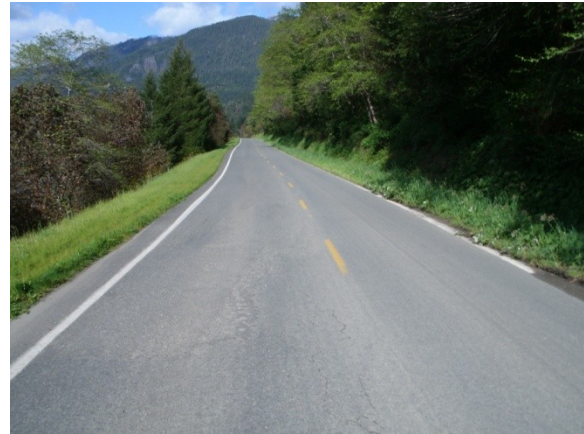
Figure 1 – Red Cap Road existing conditions
