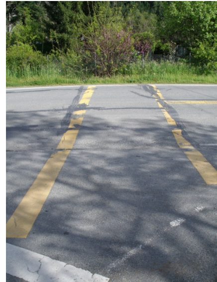
Figure 1 - Pathway on west side of SR96 looking south.
