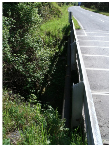
Figure 3 – Rough and Ready Bridge, south side.
