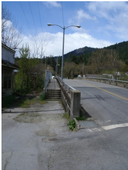
Figure 2 – Non-ADA compliant pedestrian access, east end
