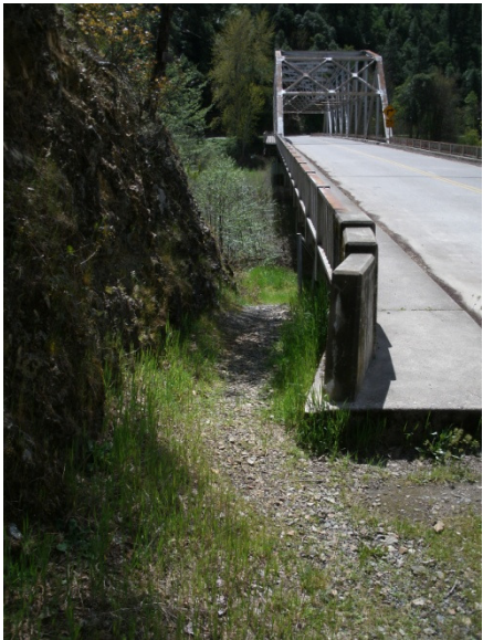
Figure 1 – Pedestrian access to trail near Curly Jack Bridge
