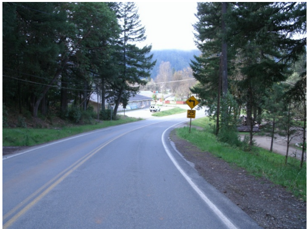
Figure 1 – Sight distance issue, southbound.
