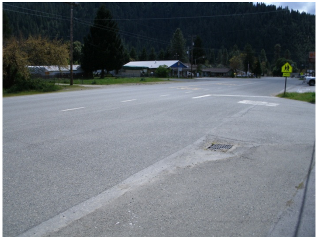
Figure 1 – Intersection looking southeast
