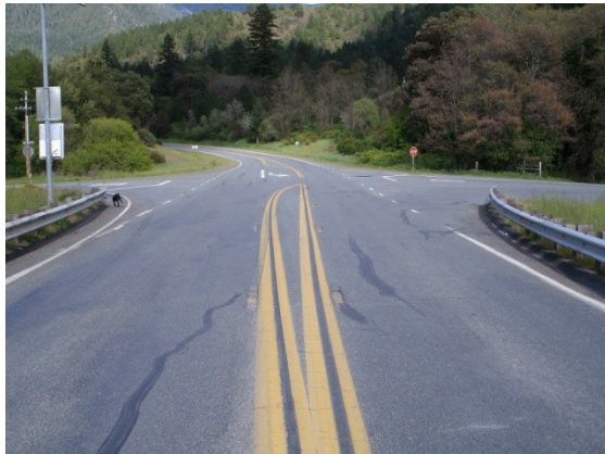
Figure 1 – State Route 96 looking east
