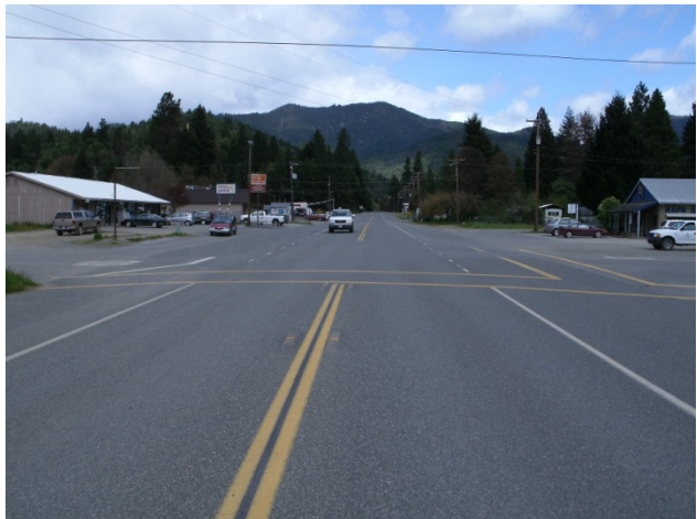
Figure 1 – Intersection looking north
