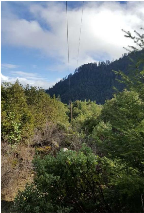
**Figure 5 Even Maintained Corridors Have Unsafe Levels of Fuels Near Lines**
