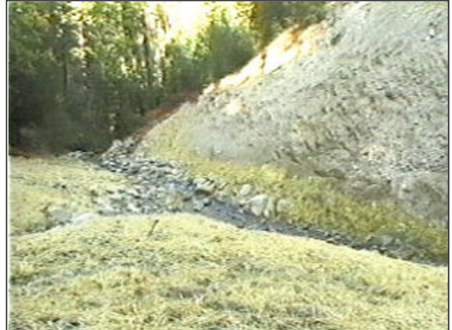
Completed RX1: note rocky outcrop on right bank and secondary channel entering from the left.
