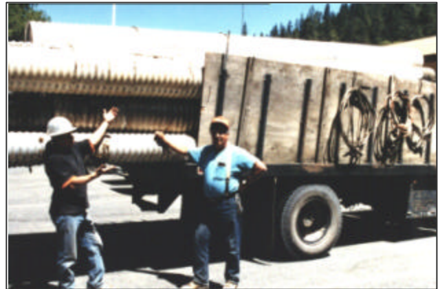
Culvert downspout being removed from the project.
