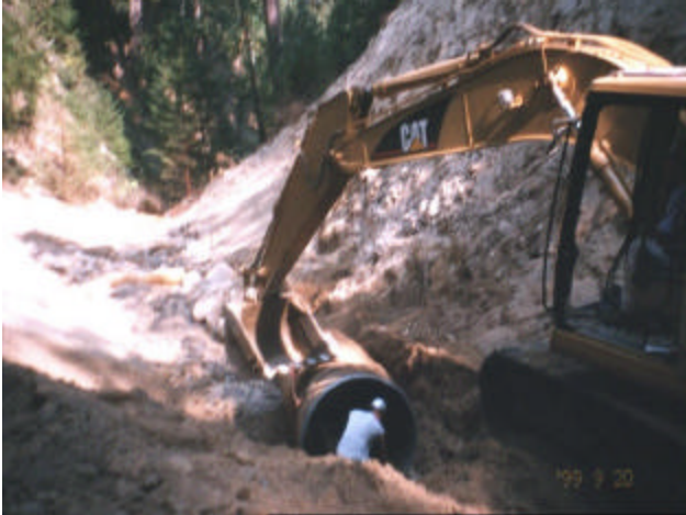
RX 1: culvert section being removed.
