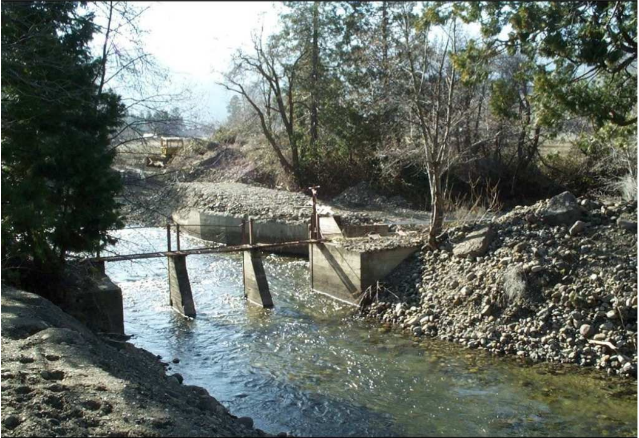
Headworks of MWCD Parks Creek diversion. (Source: water master)
