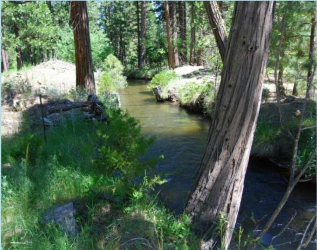
Parks Creek Diversion 183 – Looking down the Yreka Ditch from the siphon outlet. Photograph taken on 20100616 .
