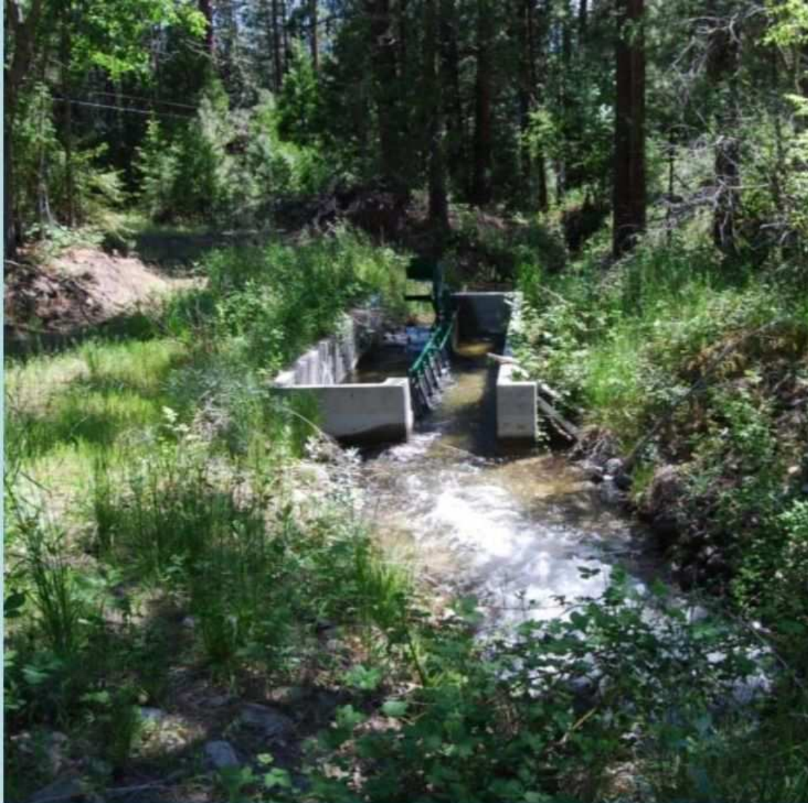
Parks Creek Diversion 182 – Looking down ditch at the DFG fish screen.
