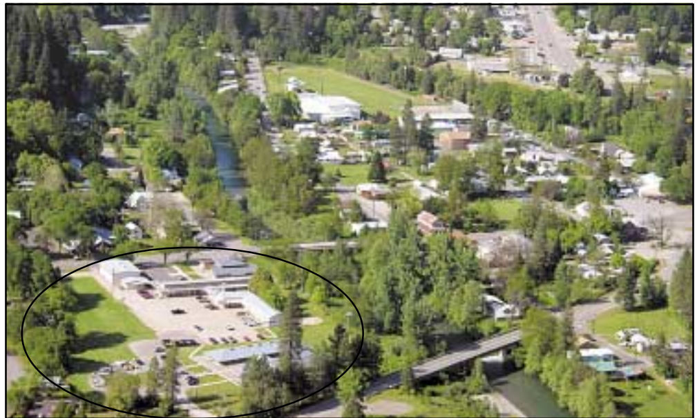
Ariel view of Happy Camp. Circled in black is the Admin Office and other Tribal buildings and structures.
