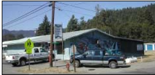
Karuk Building Center in Happy Camp
